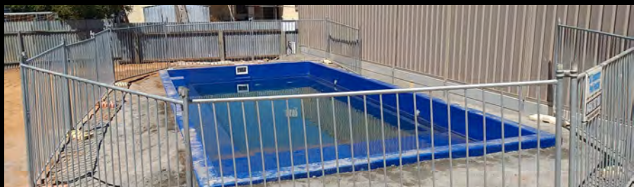
TEMPORARY POOL FENCING
